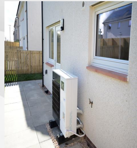
Mitsubishi Ecodan PUF & hot water cylinders
