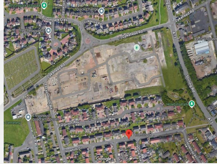
Cleared Site – 5.4ha
