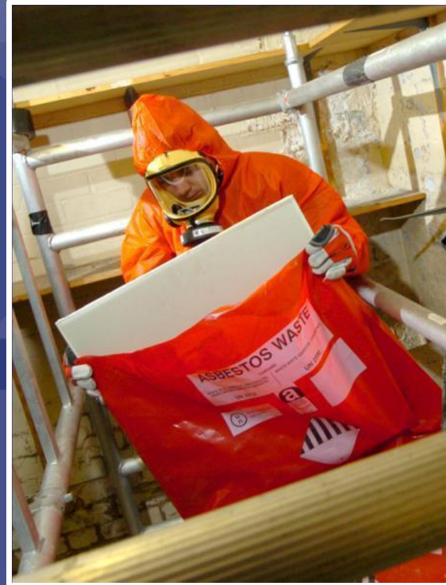
Bagging sectional asbestos lagging & AIB
