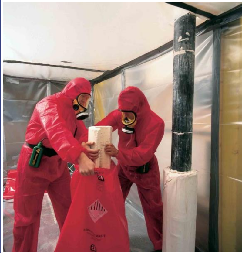
Bagging sectional asbestos lagging & AIB
