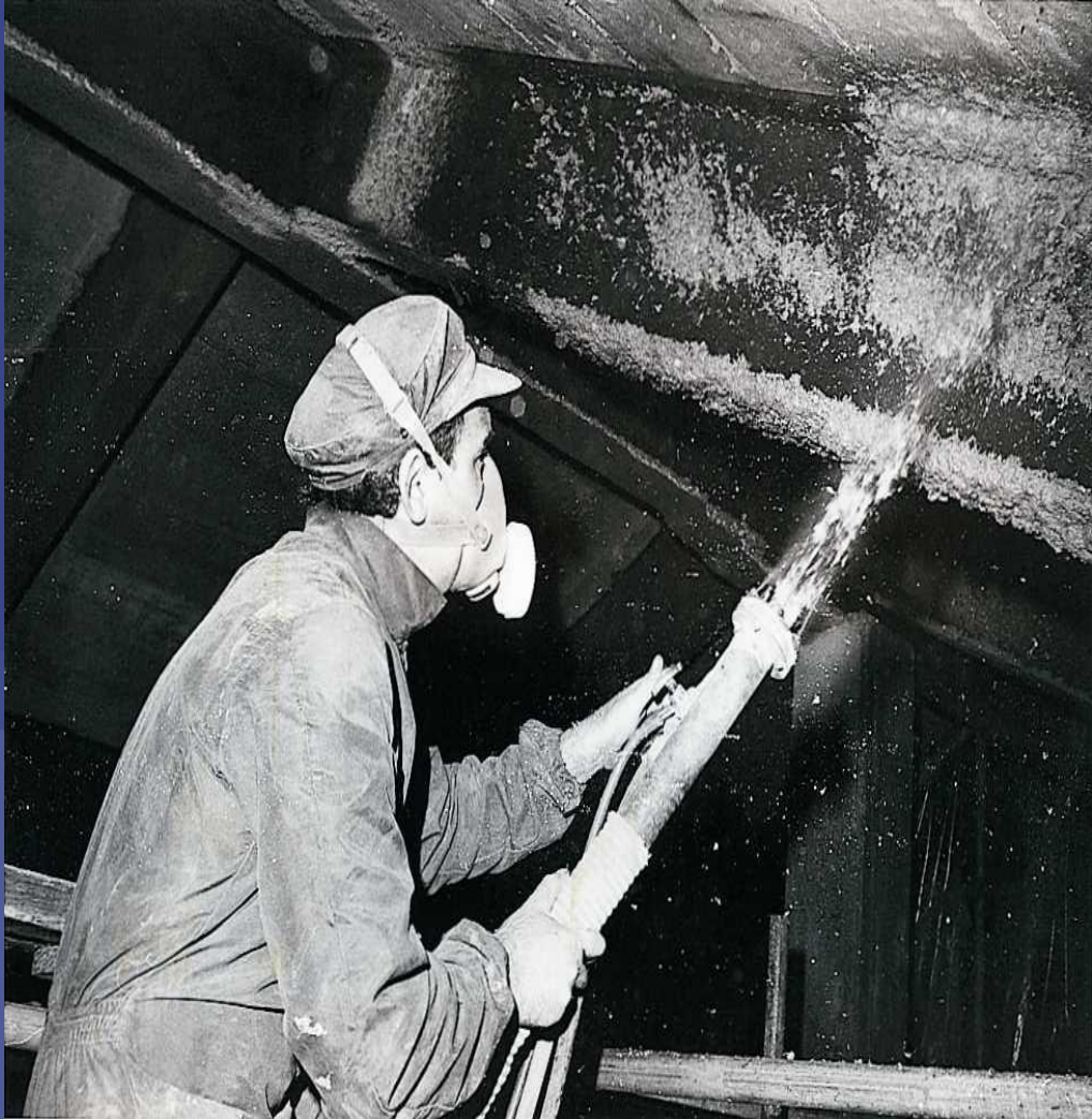
Original application of ACM Sprayed Coating
